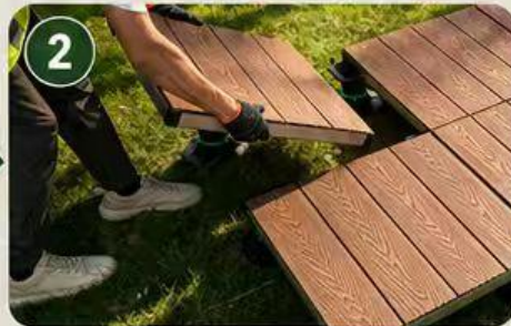
Position and connect the floor panels
